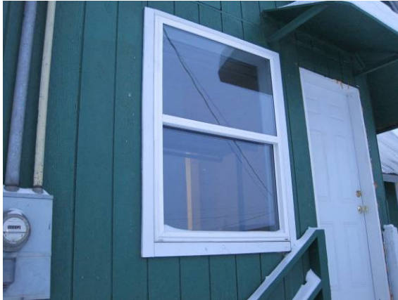
Exterior Windows in Good Condition
