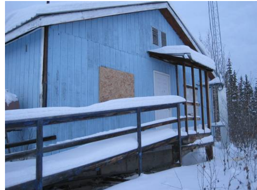
Exterior and Boarded-up Windows
