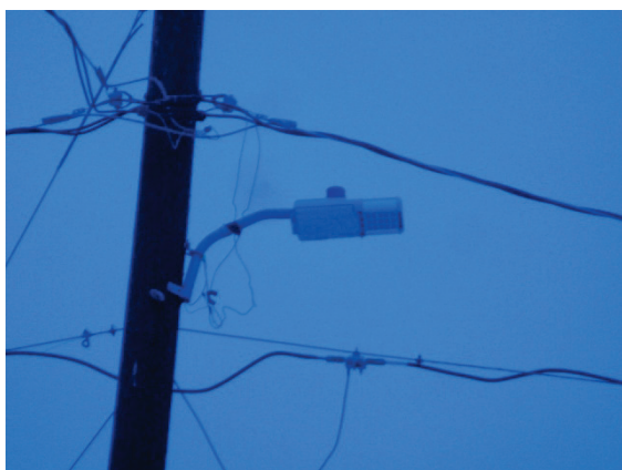
LED Street Lighting Upgrade
