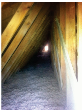
Thermal Insulation Upgrade – Addie Shewfelt Building
