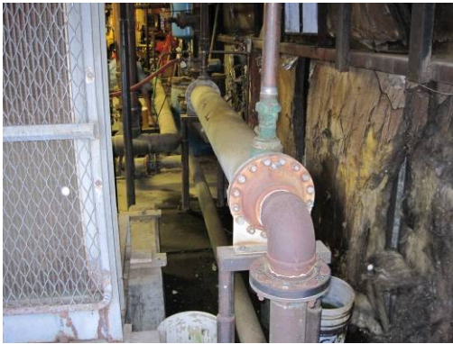
Deteriorating Insulation
