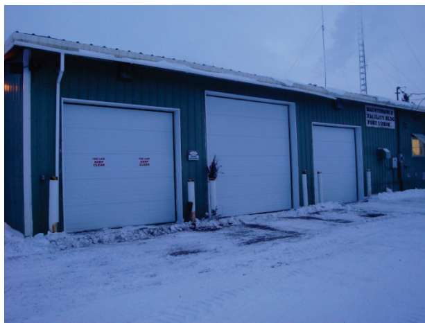
New Overhead Shop Doors – City Hall
