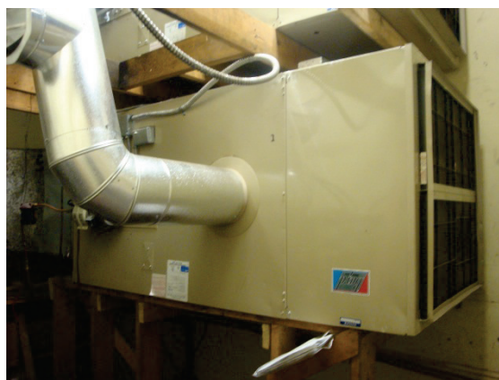
Furnace Upgrade – City Hall
