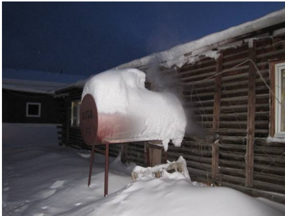
Wood Stove Vent and Storage Tank
