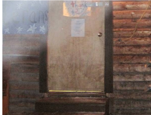
Non-Weather-stripped Door
